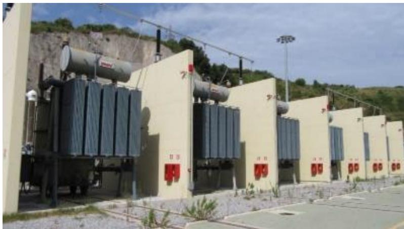
**Figure 4 . 3: Firewalls – Réactances shunt**
