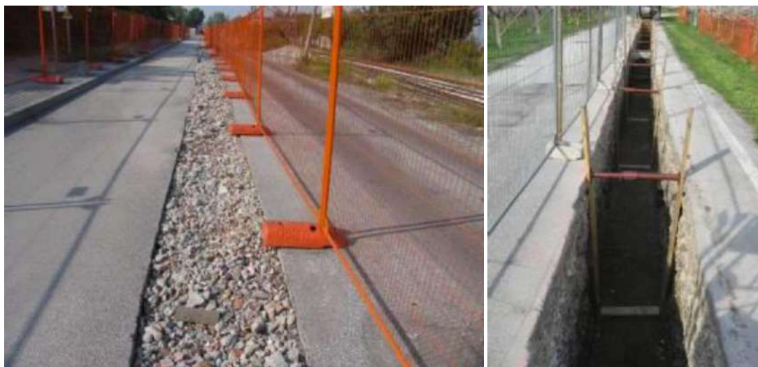
Figure 4.5: Example of cable installation on a paved road
