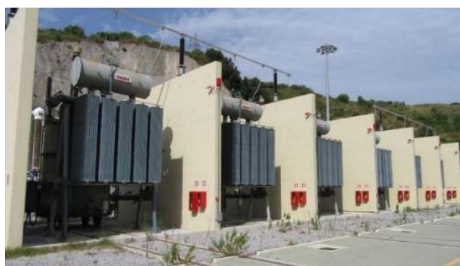
Figure 4.3: Firewalls – Shunt reactors
