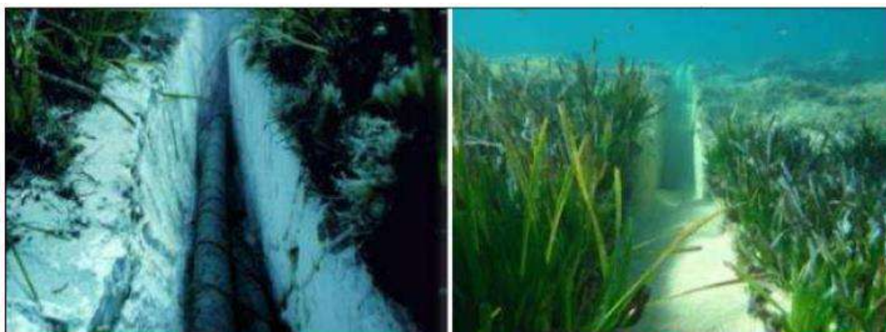
Figure 4.17: Trench over Posidonia generated with controlled floating trenching machinery
