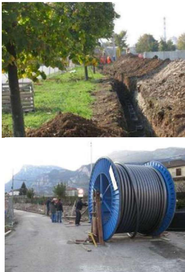
Figure 4.6: Example of cable laying in a trench
