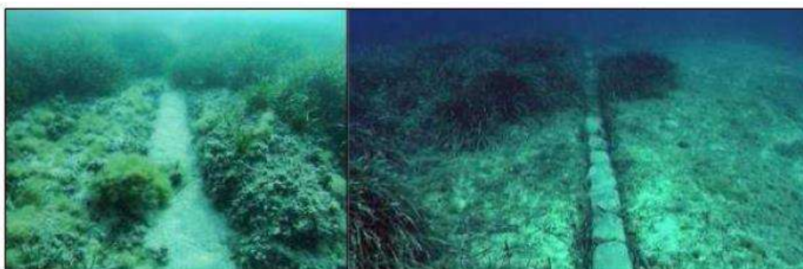
Figure 4.14: Trench over Posidonia on sand generated with a jetting machine
