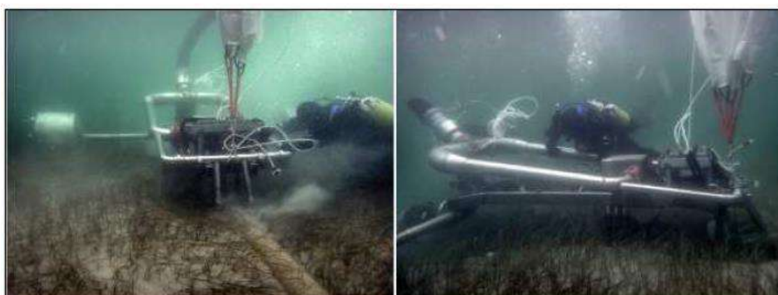
Figure 4.13: Machinery for jetting over Posidonia oceanica on sand sediments
